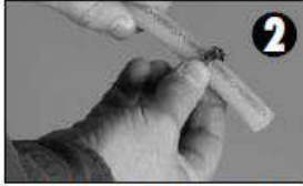
2 Slide clamp or crimp ring over tube.
